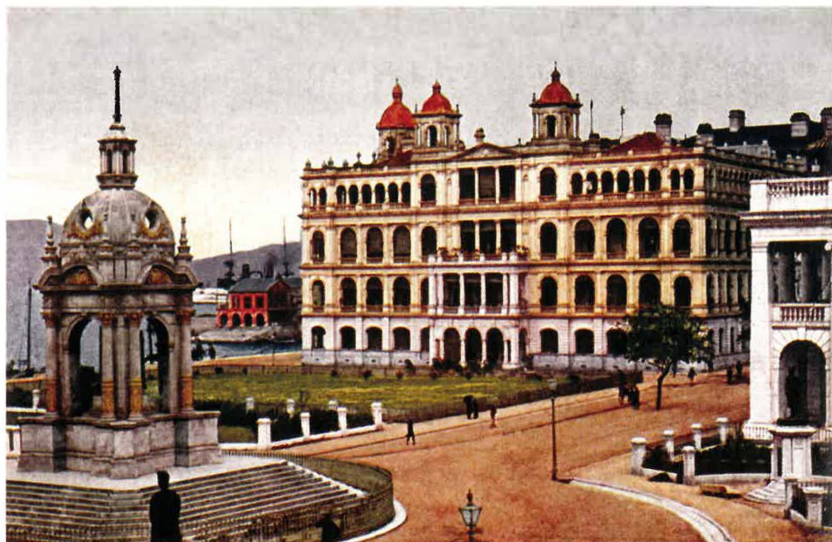
The Hong Kong Club was among the first buildings to stand on the 59 acres that CP Chater's 1890-1904 reclamation project created in Central.
